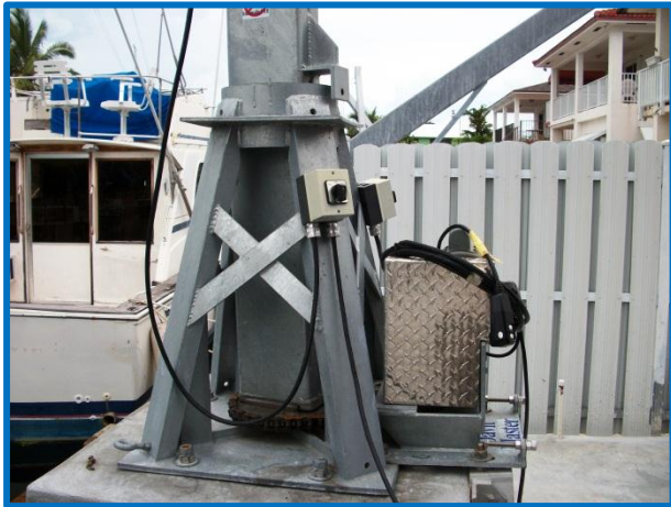
Power Pivot -concrete base
